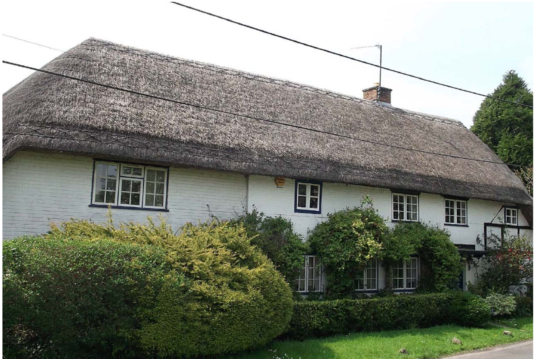
Grade II Listed Building opposite site/entrance
